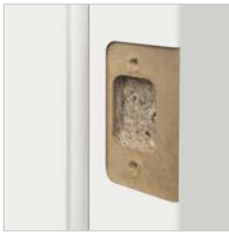
STRIKE PLATE preparation for standard 2 1/4" strike plate
